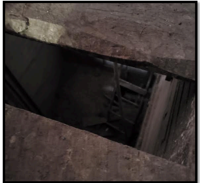
Ladder inside bin.
